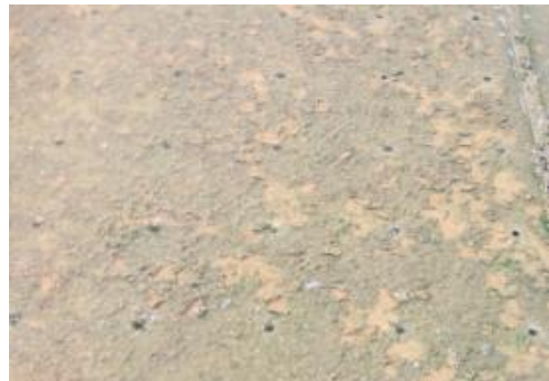
Figure 1: Dirt and biofilm on a cooling tower distribution deck is shown sloughing off after an application of a biodetergent.
